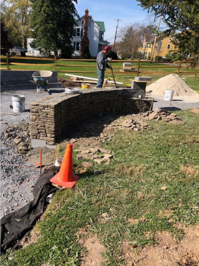
Lillard's Corner under construction
